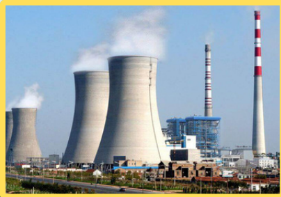
Dr. Narla Tata Rao Thermal Power station
